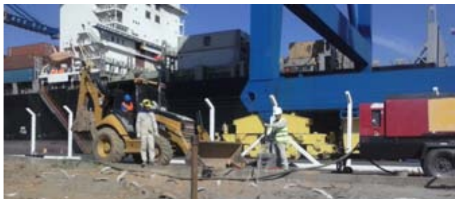
As obras de ampliação do cais, com CPR Grouting.
